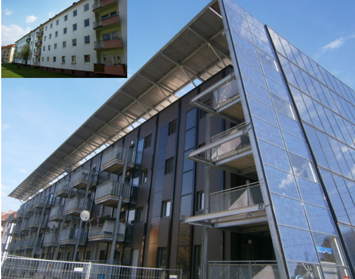
Ongoing EBC research into cost effective renovation: Kapfenberg case study – View of the existing (inset) and the renovated building (main picture). Source: AEE – Institute for Sustainable Technologies.
