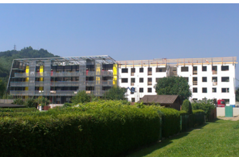
Kapfenberg case study – View of the finished renovation (left part of building) and still in renovation (right part of building). Source: AEE – Institute for Sustainable Technologies
