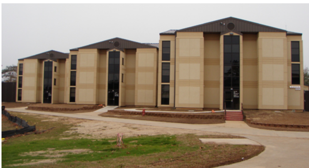
Renovation of barracks achieved a 45% energy use reduction through better insulation, improved airtightness, a dedicated outdoor air system, enclosed stairways with a vestibule and a covered atrium with increased usable space (Fort Polk, USA). Source: U.S. Army Corps of Engineers
