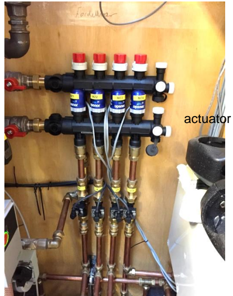
Figure 27 The heat exchangers emulating the heat emitters in a heating system (left). The actuators of the heating system (right).
