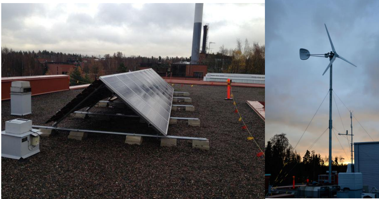
Figure 13 PV panels and micro wind turbine on the roof of the building where nZEB emulator is located.
