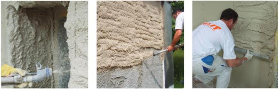
Figure 77: Application of high-performance insulating plaster on a façade.
