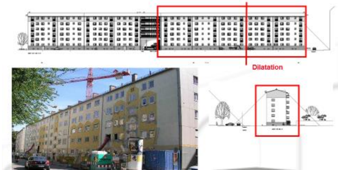
Figure 58: Building in Munich, Germany, where LOCKPLATE system was installed.
