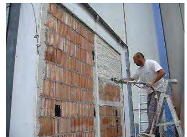
Insulating mortar projection.
