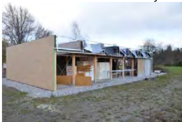
Facility during erection process
