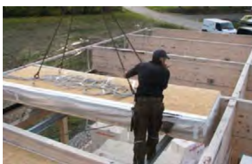
Mounting of roof assemblies
