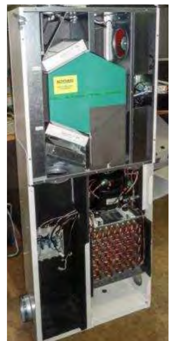
MVHR-unit with micro-heat pump (Project iNSPiRe)
