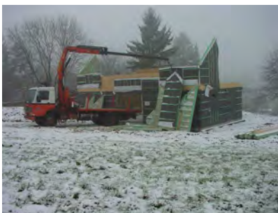
View of the facility during construction
