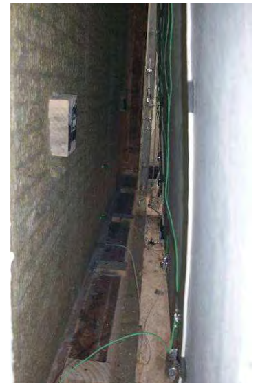
Closing the air chamber, wooden separators to maintain the air gap uniform. Thermopile cables in green.
