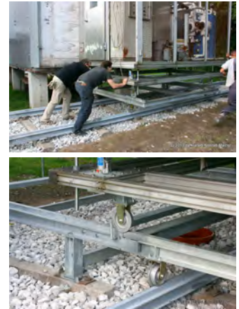
Rail system for positioning of the movable Cold-Box
