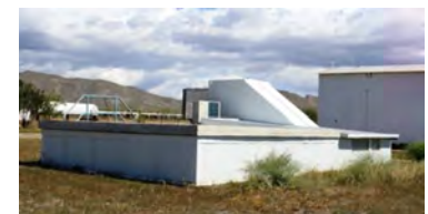
Exterior of the CETeB Test cell
