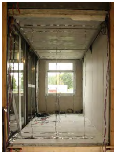
Full scale test room during construction: concrete floor and ceiling, window in SW façade, windows in room side wall
