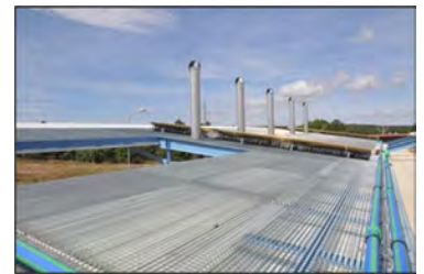
C-Ddl CEDER. Radiant night cooling system
