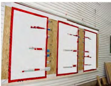
Test bays nearing completion.
