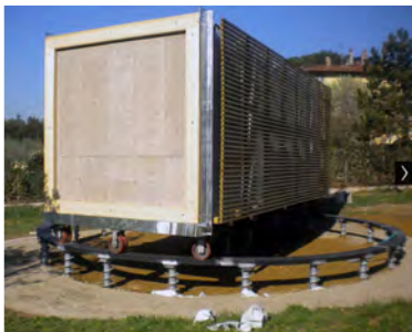
View of the circular platform base, connected to the ground with screws Krinner type.
