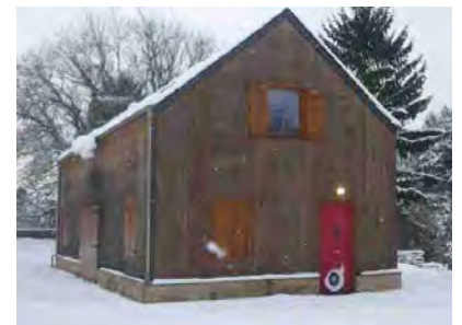
Blower-door test conducted on the building
