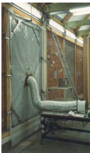
Inside view; an airtightness test is performed on one of the facade elements.
