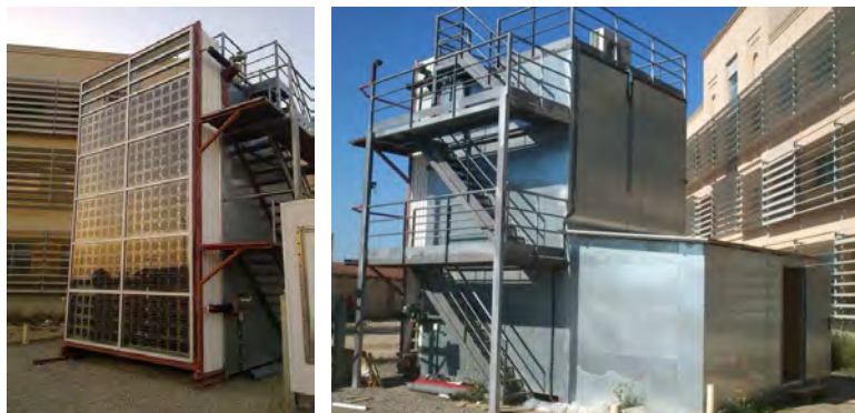
Figure 1. LOT test facility. Front and rear view.
