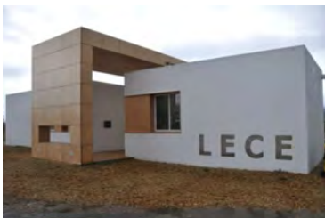
Monozone building. North face
