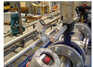
Test of circulation pumps.
