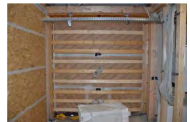
Research regarding fungi growth in building envelopes made in timber construction
