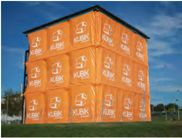
Picture of the building with no elements in the façade (with no configuration)
