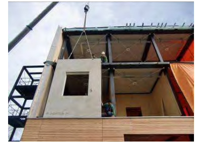
Prefabricated concrete façade element, developed with Norten-pH
