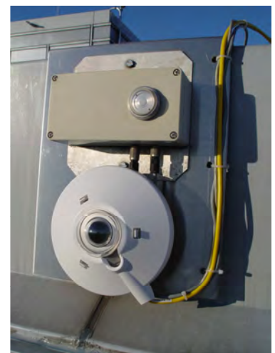
Measurement of the illuminance at the south facade of VERU
