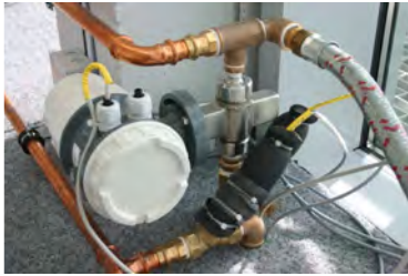
Magneto-inductive flow meter for determining mass flows in heating and cooling circuits.
