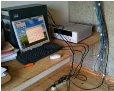
View of the Data Acquisition Unit placed in the Service Room.
