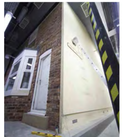
The building following a deep retrofit project, illustrating the flexibility of the property
