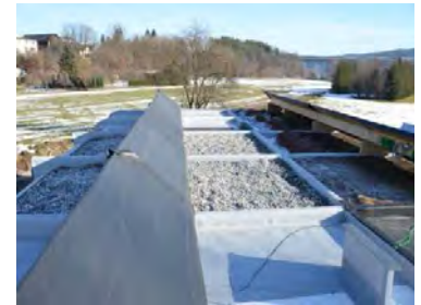
Investigation regarding roof shadings
