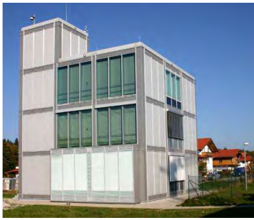
South-west view of the VERU test building.
