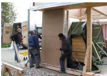
Mounting of wall assemblies
