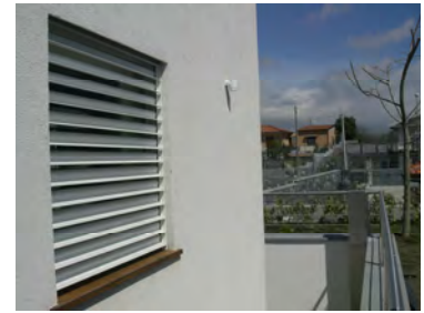
External movable solar shading blinds, automatic controlled. The actual position of them will be logged at each time step.
