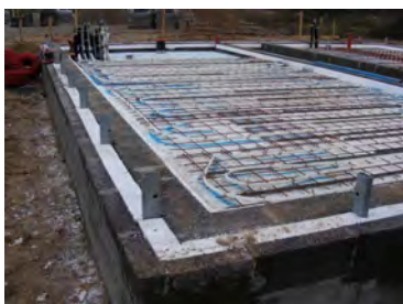
Floor heating in the ground floor during construction of EnergyFlexHouse.
