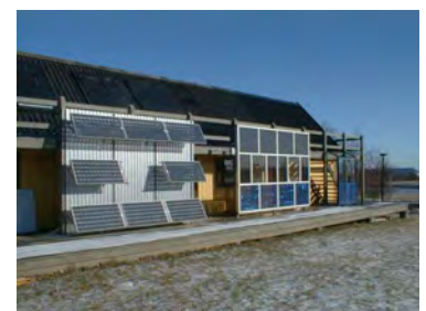
Test of pv systems.
