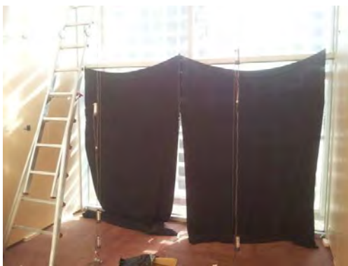
Figure 5. Mounting the inner solar protection
