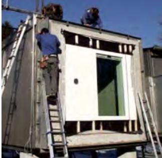
Mounting of test component (Project INTENSYS)
