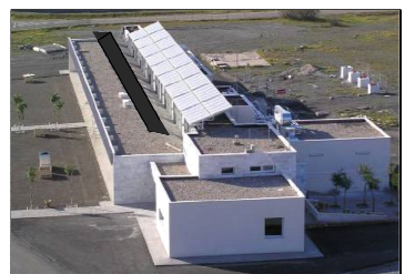
The PSE ARFRISOL C-DdIs: Office building prototype in occupancy conditions
