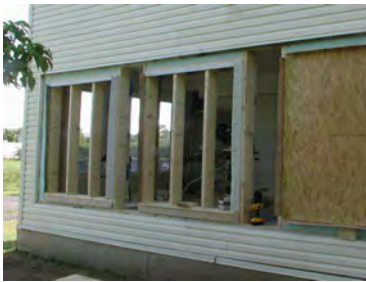
Three test bays in preparation.
