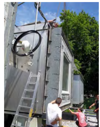
Mounting of test component (Project water:solution)
