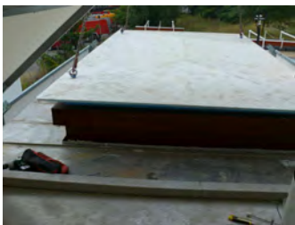
Removing the calibration roof from ILARGI.
