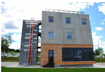
Eastern façade of KUBIK
