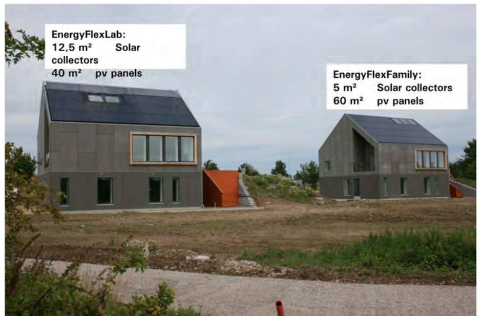
Figure 3: The solar collectors and pv panels of the two EnergyFlexHouses. Approximately 20 m 2 pv is needed for the electric vehicle.
