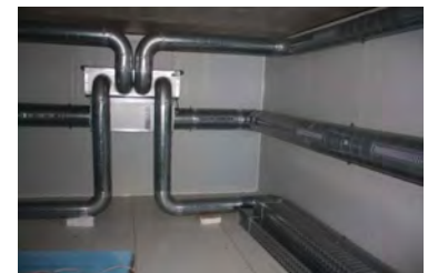
Interior of the CETeB Test cell
