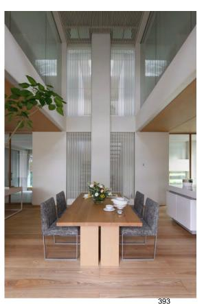
Louver-type Shutter to shade excessive solar heat gain during summer
