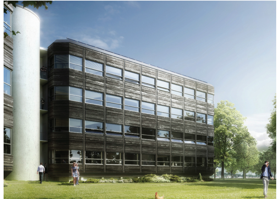
Power House Kjørbo, Norway. Copyright: Snøhetta
