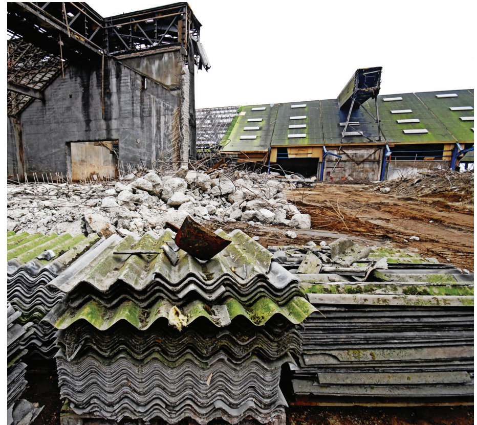
Disassembly of industrial complex. Copyright: Colorbox
