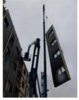
Figure 4: prefabricated façade element
