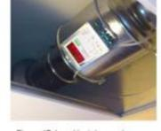
Figure 17: LeanVent damper in place on an air inlet duct to reduce energy consumption
