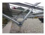
Figure 11: renovated flat roof with scatfold for the mounting of the photovoltaic panels
