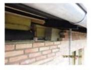
Figure 7: New insulation and new bricks near the roof
