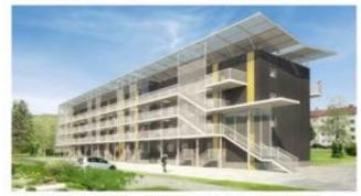
Figure 13: rendering with renovation concept for the roof (solar panels)
