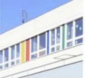
Figure 14: Row of windows (2<sup>rd</sup> floor) after renovation separated by colored plastic panels.
