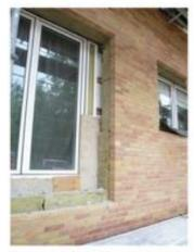
Figure 8: The new insulation and new windows almost in place
