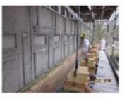
Figure 9: New 190 mm insulation plus exterior solid standard bricks in the construction phase - shown with scaffolding
