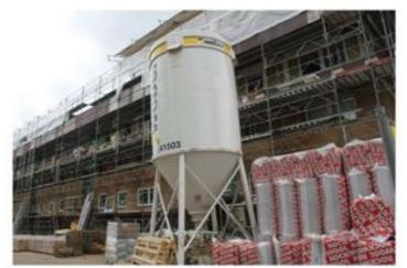
Figure 21: Insulation material waiting to be installed at the foot of the scaffolding
