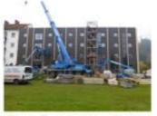
Figure 7: assembling of the prefabricated façade elements
