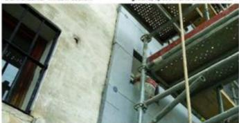
Figure 16: Installation of facade insulation, 6cm extruded polystyrene.
