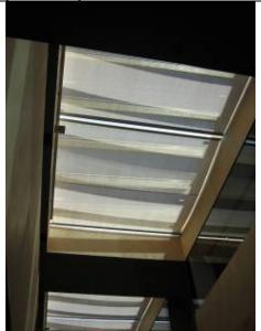
This picture shows the internal shading device in the atrium. The shading is activated when the temperature in the cavity is 40°C.
