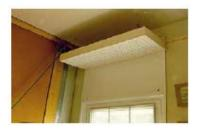
by a controlled grill at the inlet side. Climate room measurements showed that the incoming air in the office rooms during wintertime could cause thermal comfort problems, due to a fall of cold air just behind the facade. The flow of cold air at floor level would cause draught complaints. Based on extensive tests the addition of a perforated shelf with 100 mm borders under the inlets was added to the design.
