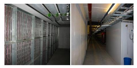
Filter at air intake in culvert (left) – low pressure drop. Storage tank for solar DHW is place in culvert (right). The culvert surfaces are painted.
