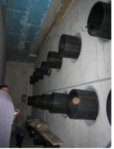
The picture shows the ducts through which the air is let into the basement area where the air is preheated or precooled.
