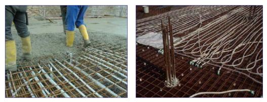
Figure 3-24 Concrete lying on the reinforcement grid with attached pipes
