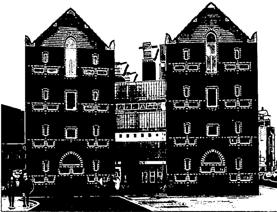
Figure 4.1 DeMontfort University Lecture Hall [Photograph Courtesy of BRE, UK]
