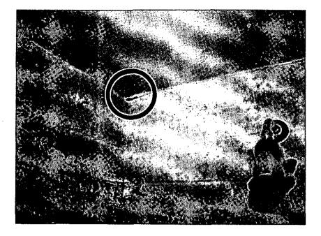
Figure 8: View to the north-west corner of the bathroom with PT100 glued against the coldest spot of the wall
