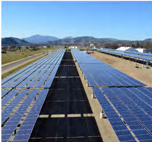
Solar panel arrays form a canopy at a construction site in Fort Hunter Liggett, California. The construction site is for phase one and two of a solar microgrid project at the installation, managed by the U.S. Army Corps of Engineers Sacramento District. Along with energy production, the panel arrays provide shade for the majority of the post's vehicles. Fort Hunter Liggett is one of six pilot installations selected by the U.S. Army to be net zero energy, meaning the installation will create as much energy as it uses. (Photo Credit: U.S. Army, John Prettyman)
