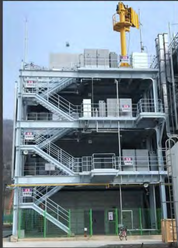
Bundang, South Korea Power Tower Installation
