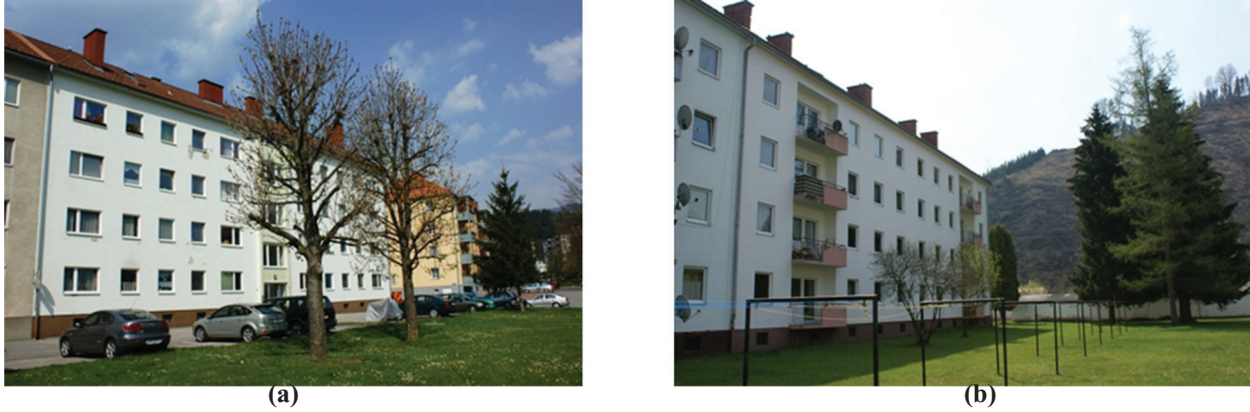
Figure 1 Views of the Austrian case-study building from (a) east and (b) west.
