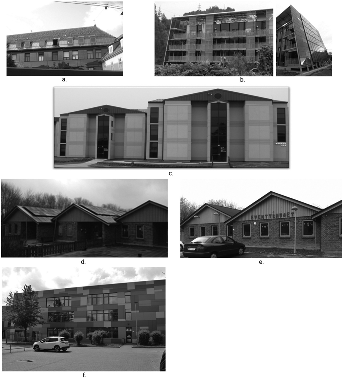
Figure 1 Example of DER projects: (a) Renovation of the medieval Franciscan monastery in Graz, Austria—zero energy building (AEE INTEC and Nussmüller Architekten ZT GmbH 2015). (b) Renovation of a residential building in Kapfenberg, Austria—85% site energy use reduction (AEE INTEC and Nussmüller Architekten ZT GmbH 2015). (c) Renovation of VOLARM barracks at Fort Polk, Louisiana—one of 30 barracks renovated to 50% site energy use reduction. (d–e) Renovation of kindergartens in Denmark (Class 1 2014). The primary energy consumption has been reduced from 71 to 33 kBtu/ft 2 /y (224 to 103 kWh/m 2 /y). (f) Renovation of a school campus in Aachen, Germany. The primary energy consumption has been reduced from 76 to 25 kBtu/ft 2 /y (240 to 78 kWh/m 2 year).
