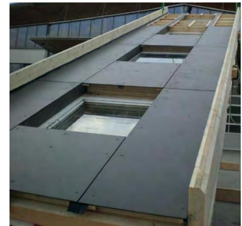
Instead of conventional insulation systems the facade in this project is covered with large-sized active and passive facade elements.
