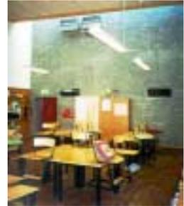
*Classroom showing supply vents half way up wall, and exhaust vents at top*
