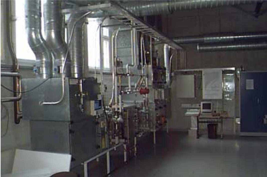
Figure C5. An overview of the demonstration system. The air-handling unit is on the left and the BEMS is on the right.
