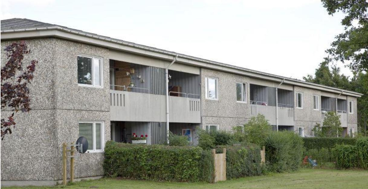
**Figure 10.** Typical prefabricated concrete building. Source: <http://www.kildeparken2020.dk/>
