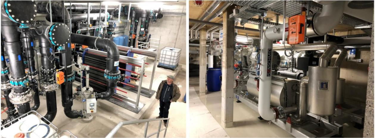
**Figure 52.** Right: Lake-water pumping station. Left: 1 MW Heat pump. Source: Corporation Weggis.
