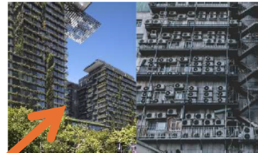
Figure 3: Cool wall use at One Central Park, Sydney (left) compared with maladaptive retrofitted air conditioning (right).
