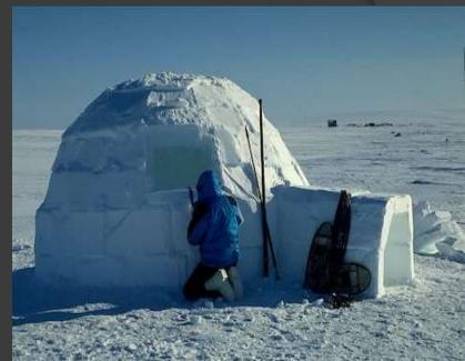
Made of ice bricks with thickness of about 500mm. The indoor temperatures can be maintained at above  $-5^{\circ}$ C when the outside temperature is  $-30^{\circ}$ C.
