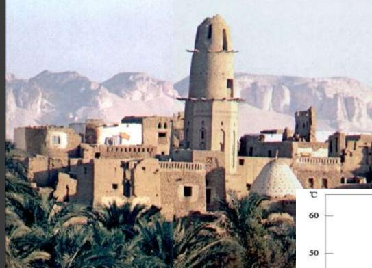
Brick thickness is more than 400mm. Due to the big thermal mass, indoor temperature difference in a day is less than 6°C, while outdoor temperature difference is more than 24°C.
